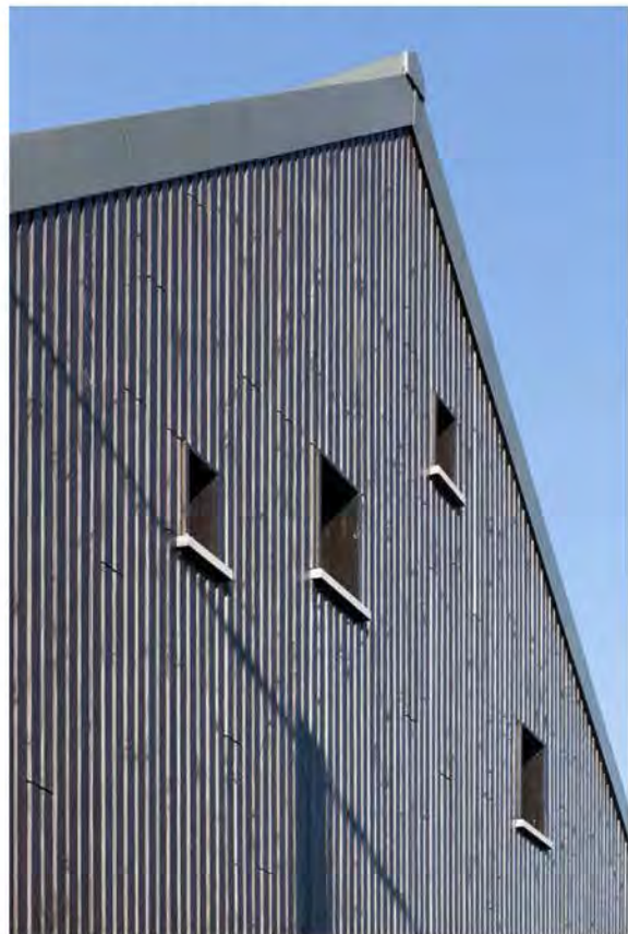
Chieveley by Gresford Architects
