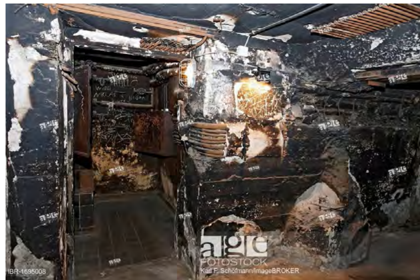
Figure 1: Tempelhof bunker fire damage
