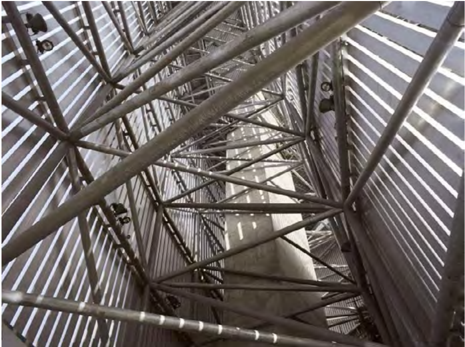
Figure 5: Imperial War Museum North, internal view of airshard Daniel Libeskind's Imperial War Museum North includes the 'airshard' an indoor/outdoor space clad in extruded box-section planks and finished with a perforated metal flooring. The building is intended to disorientate the visitor.
